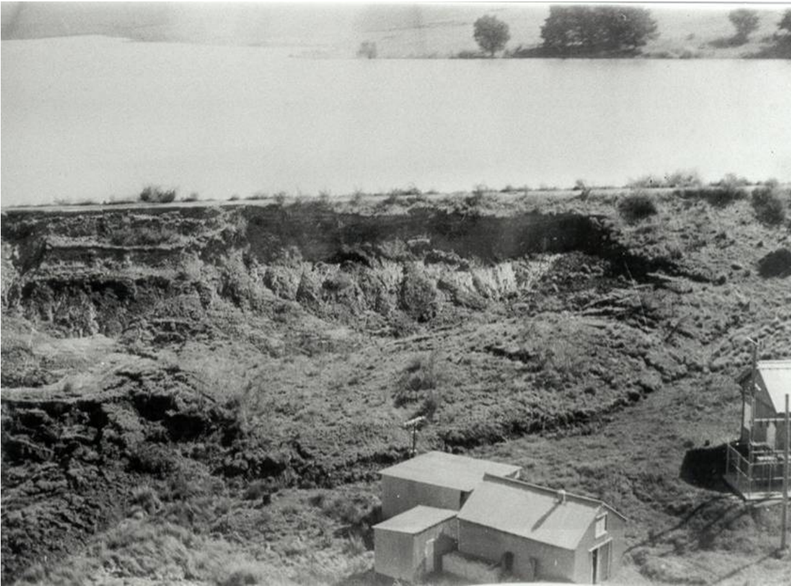
Figure 2: Spring Creek Dam, 1966 Downstream Slope Failure
