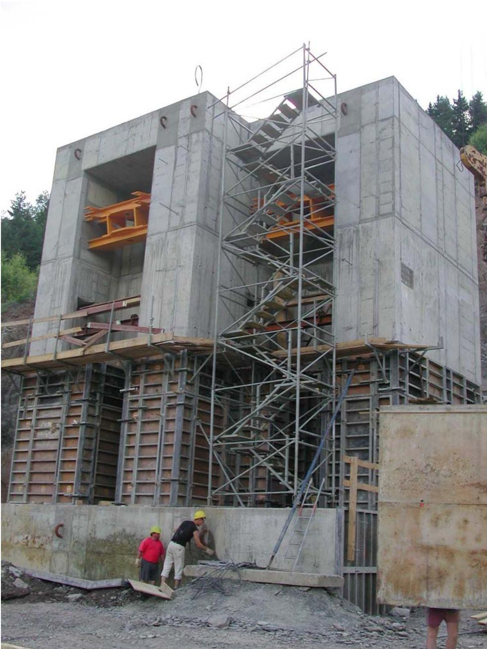
Fig.: 9 Cable crane – installation fixed point
