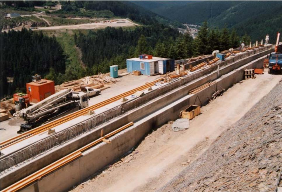
Fig.:10 Cable crane – rail track installation for the counter carriages
