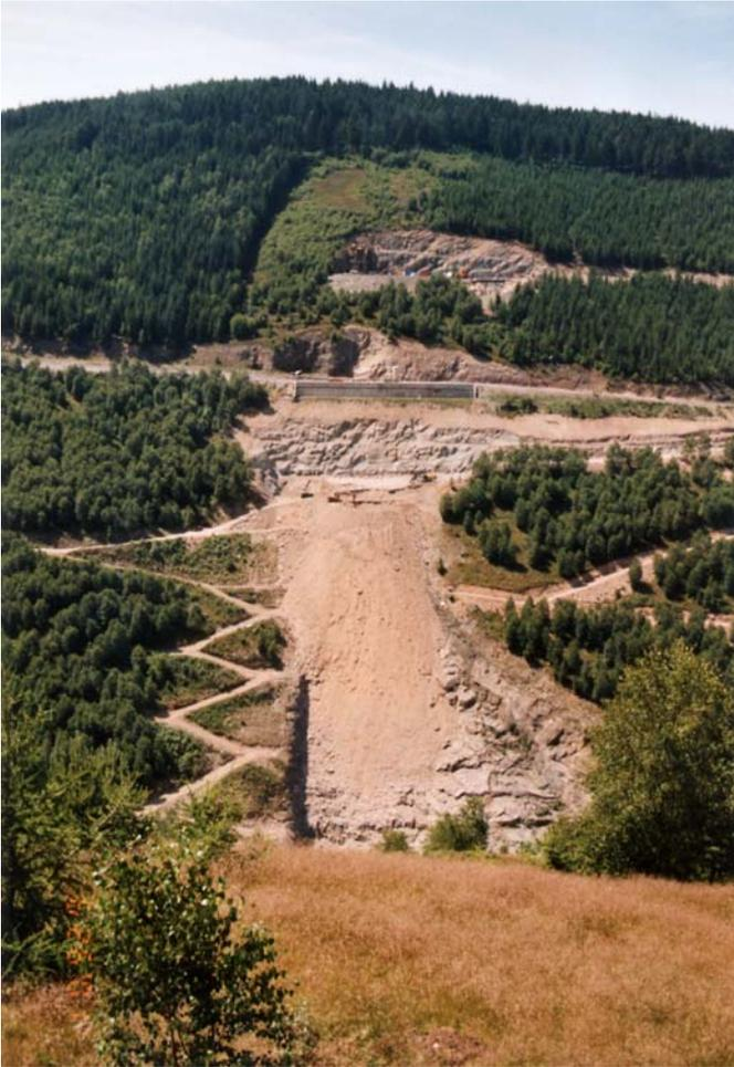
Fig.: 8 *Pit excavation left abutment*
