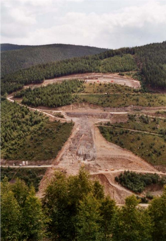
Fig.: 7 *Pit excavation for the concrete dam (right abutment)*
