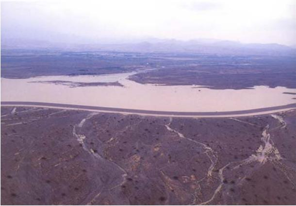
recharge dams have been built in many arid countries. Though the storage of rainwater in surface reservoirs by dams has the disadvantage of increased evaporation losses, it brings the advantageous possibility to manage the recharge process by operation of the dam facilities (fig. 1).
