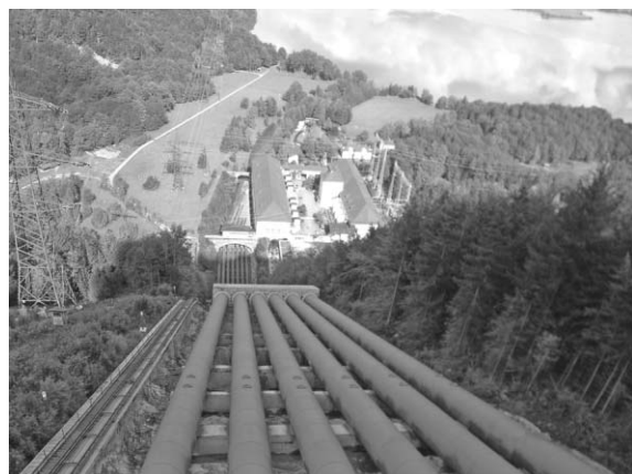
Fig. 1. Walchensee hydropower station
