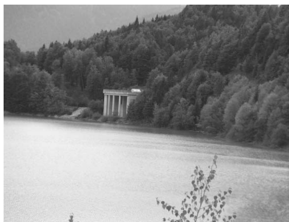
Fig. 4. Sylvenstein overflow structure known as the Sylvenstein Temple
